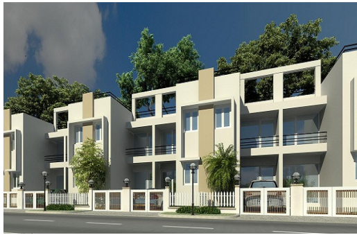
SARE KOLATHUR, CHENNAI (VILLA)
