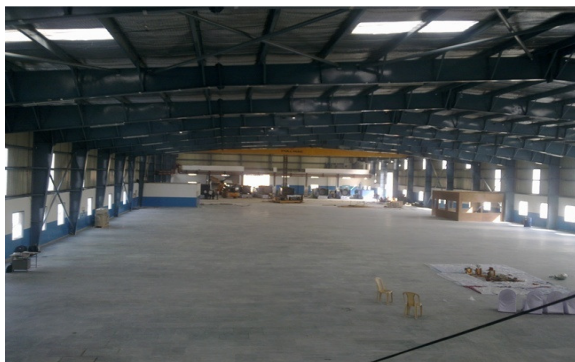
PLANT FOR INJECTION MOULDING AT G. NOIDA (ONS INFOTECH)
